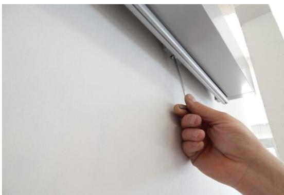
8. Lock the cassette in brackets by tightening the screws.
