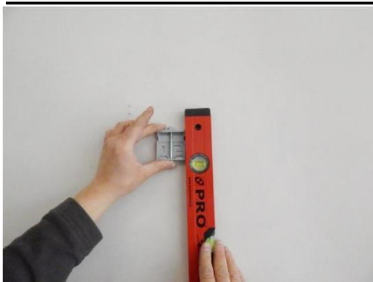
2. With spirit level mark vertical level of the bracket axis.
