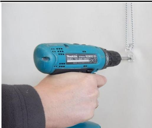
10. Stretched chain has to be fixed to the wall by adjusting the added safety element – on the height 150cm from the floor minimum. If necessary adjust the chain length.
