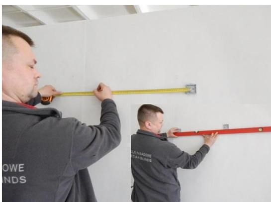
4. Measure and mark installation spot for remaining brackets. Use spirit level to mark vertical alignment.
