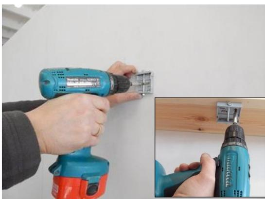
3. Install first bracket to the wall / ceiling (detail – ceiling installation)
