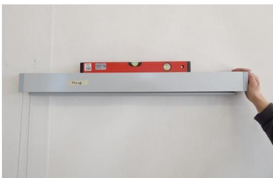
9. Check horizontal level of the installed cassette.
